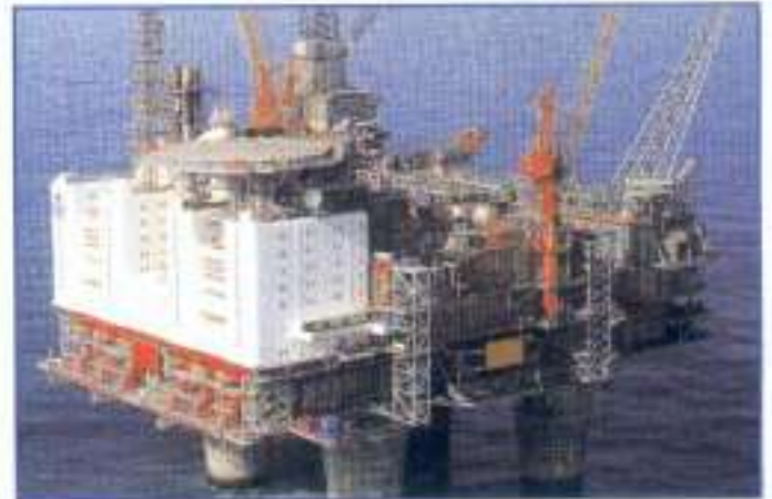
▲ Off-shore oil producing platforms
