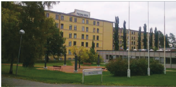
Pikonlinna Hospital, protected with SEM-SAFE® high-pressure water mist system from Danfoss.
