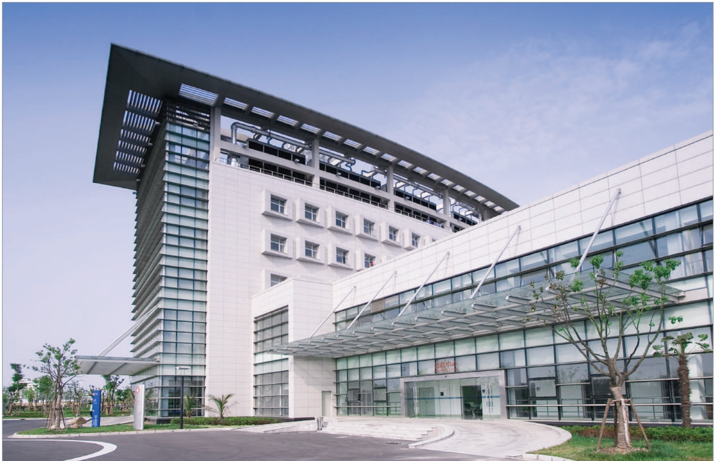
Shuguang Hospital in China, protected with SEM-SAFE® high-pressure water mist system from Danfoss.
