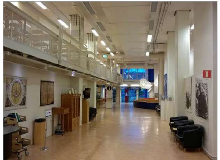
The library at Lund University which is fully covered with SEM-SAFE® high-pressure water mist system for fire fighting from Danfoss.
